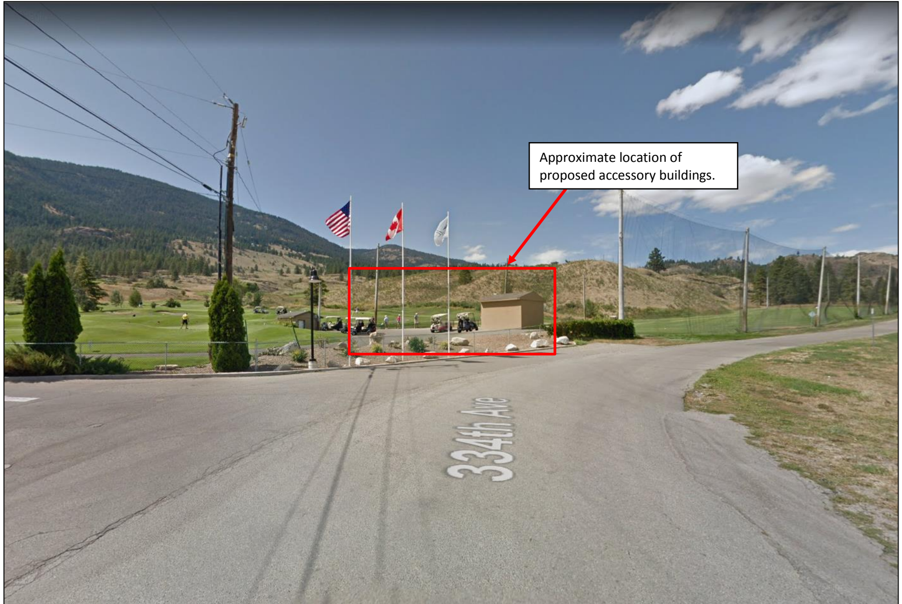
Attachment No. 1 – Site Photo - Location of Requested Variance (Google Streetview - 2012)
